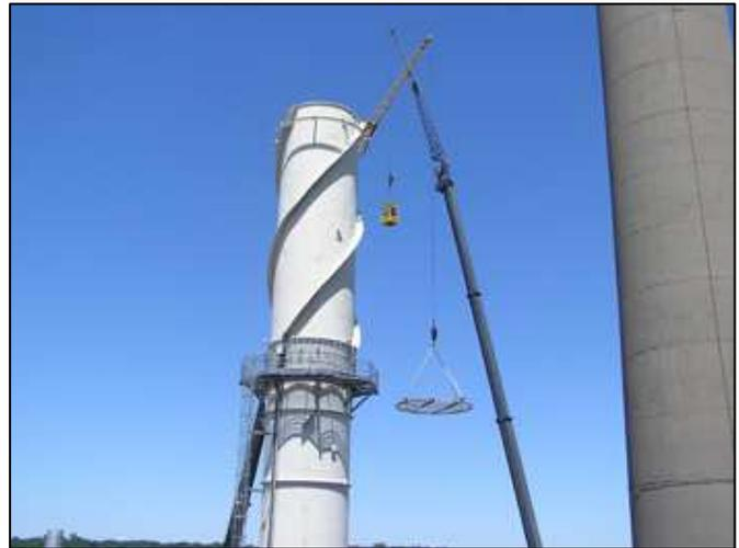
*Installing the screen. The small yellow 'box' contains two men who will weld the screen (at right) once it is placed on the top. The falcon's stack is to the right.*
