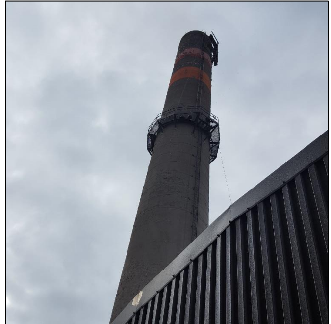
Stack repairs. The nestbox is around the stack on the first catwalk. The temporary scaffold on top was erected for stack repair.
